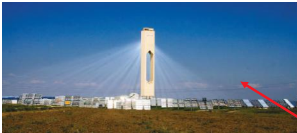
SNL Solar Tower
